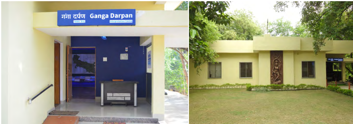
Ganga Darpan after renovation and fabrication
