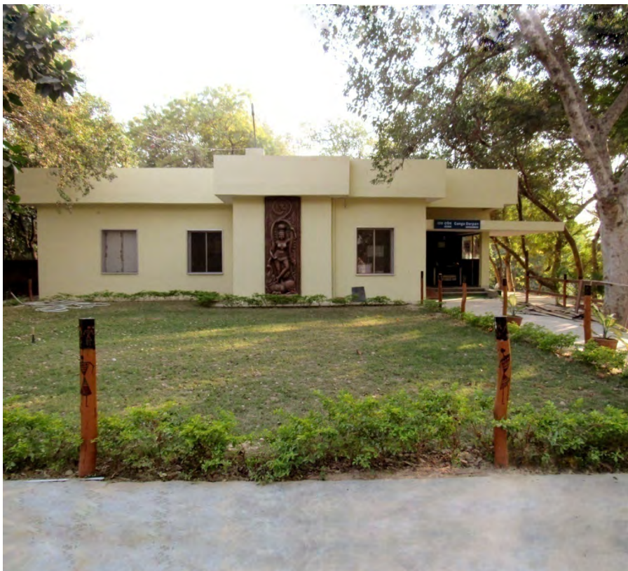
Interpretation centre building in Sarnath after renovation
