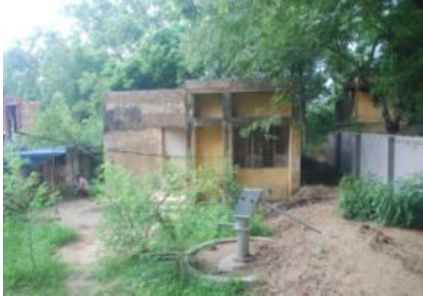
Building prior to renovation
