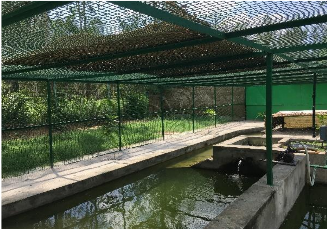
Enclosures prior to preliminary upgradation
