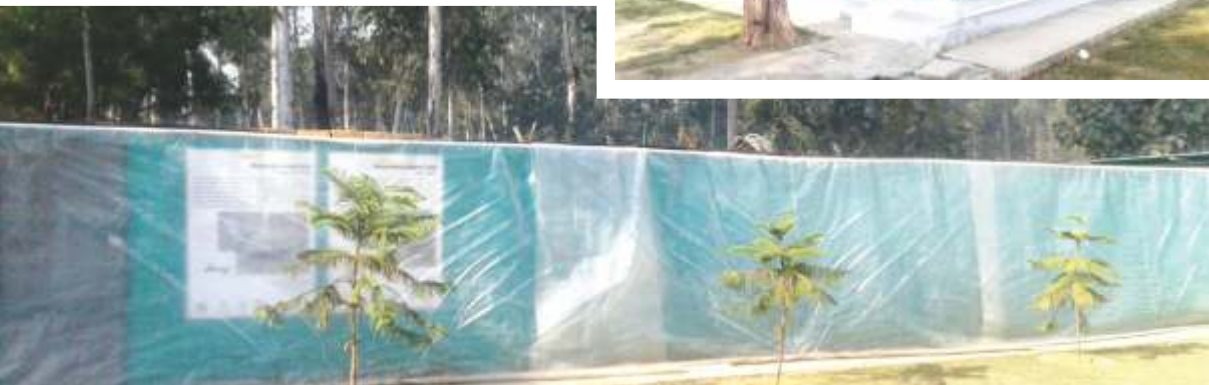
Covering of enclosures with tarpaulin to prevent temperature drop during night
