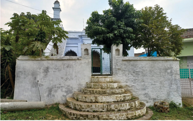
Figure 11 : Mosque, Karauli Bhudhkar, Dalmau tehsil Source: Primary survey by AH Division, INTACH Team
