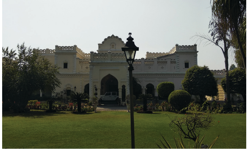
Figure 24 : Arkha Kothi, Arkha, Unchahar tehsil Source: Primary survey by AH Division, INTACH Team
