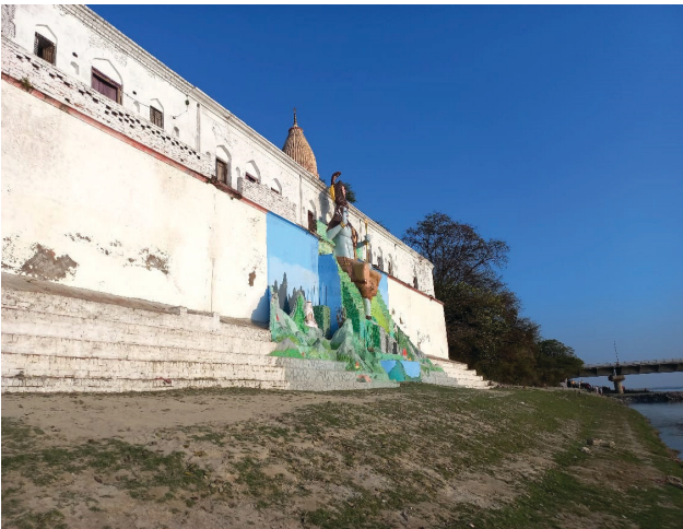
Figure 21 : Bada Math facing Ganga, Dalmau Source: Primary survey by AH Division, INTACH Team
