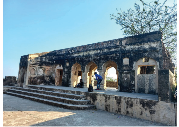
Figure 8 : Historic structures still existing within Raja Dal's fort. Source: Primary survey by AH Division, INTACH Team
