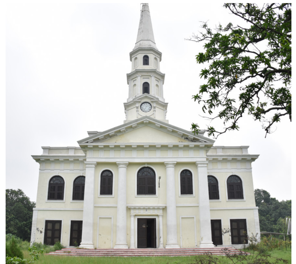
Figure 47: St. John's Church Source : Primary Survey by AH Division, INTACH Team
