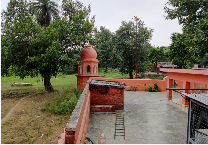
Figure 30: Pandeshwar Temple Source: Primary survey by AH Division, INTACH Team
