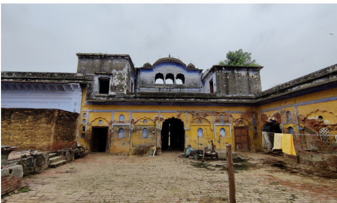
Figure 32: Diwan Khana, Behsuma Source: Primary survey by AH Division, INTACH Team
