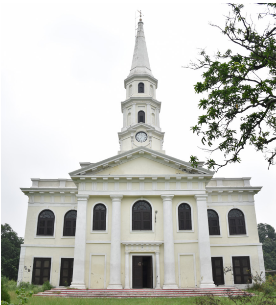
Figure 2: St. John's Church, Meerut Cantonment Source: Primary survey by AH Division, INTACH Team
