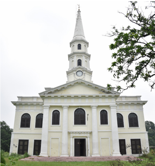
Figure 56: Front facade of St, John's Church. Source : Primary Survey, INTACH team
